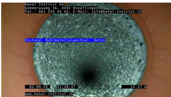
11, 00:06:54, 12.35m Rohrmaterialwechsel: Beton
