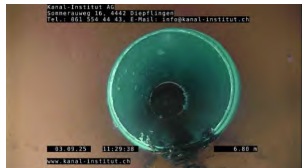
4, 00:01:22, 6.80m Rohrmaterialwechsel: Polyvinylchlorid
