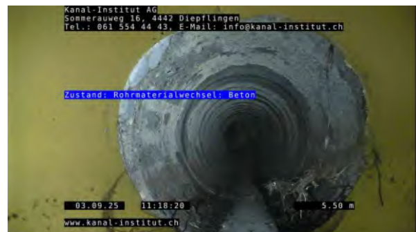
4, 00:01:53, 5.50m Rohrmaterialwechsel: Beton
