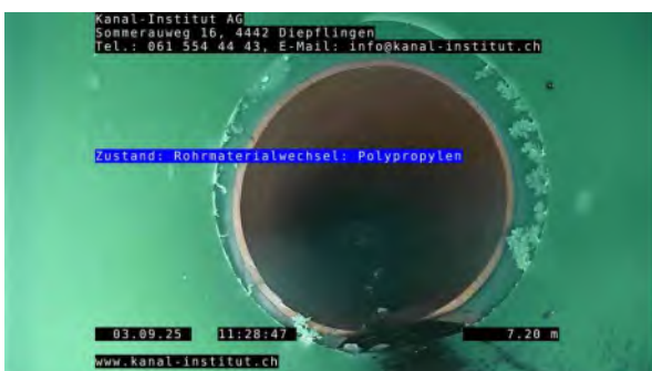
5, 00:01:02, 7.20m Rohrmaterialwechsel: Polypropylen
