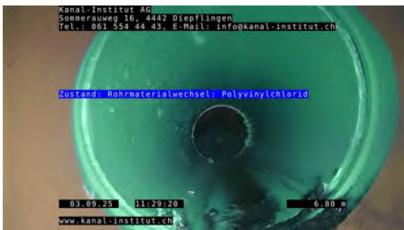
3, 00:01:22, 6.80m Rohrmaterialwechsel: Polyvinylchlorid
